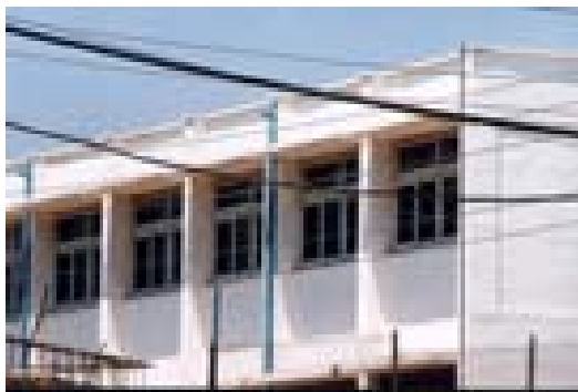
Photo (53) Cantilever Shading Elements in School Building – Al-Jalazon Refugee Camp
