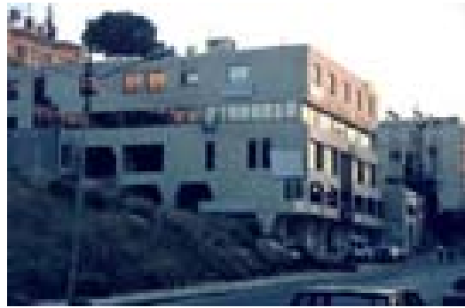
Photo (29) Commercial Building - Nablus
