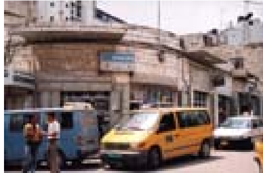
Photo (28) Linear Shops – Ramallah One Storey
