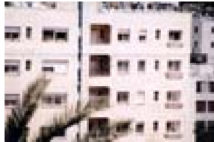
Photo (43) Residential House Openings
