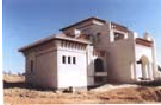
Photo (60) General View
