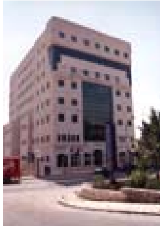
Photo (45) Curtain Walls
