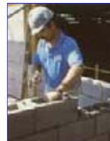
The standard concrete block is a rectangular 8X8X16-inch unit (20X20X40 cm) made mainly of Portland cement, gravel, sand, and water. The concrete mixture may also contain ingredients such as air-entraining agents, coloring pigment, and water repellent. During the manufacturing process, a machine molds moist, low-slump concrete into the desired shapes. These blocks then undergo an accelerated curing process at elevated temperatures inside a special chamber
