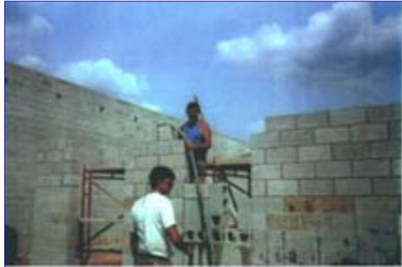
ACC is reasonably frost and sulfate resistant, allowing it to be used around the world in all climatic zones and for a wide range of applications. When it is used on the exterior, ACC is normally protected by stucco or other protective coatings. ACC also is an inorganic material, making it 100 percent termite and vermin proof and resistant to rotting and mold
